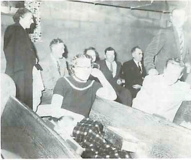
Basement of new church - 1957.
